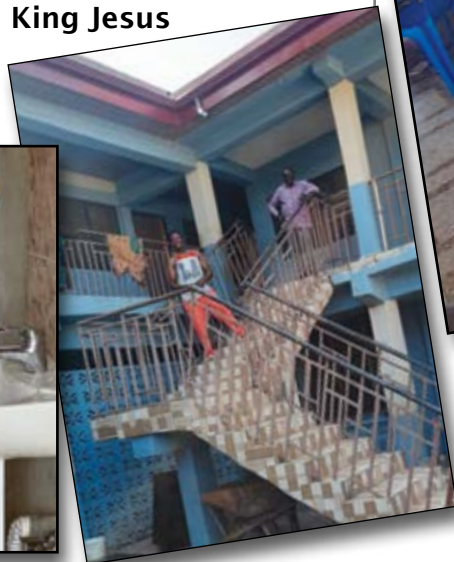
The newly tiled outdoor staircase.
